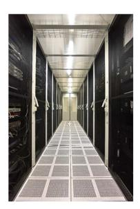
CL's Group main data center is about 450 m2 with 120 kW of net IT load and is designed to handle all the functions of the Bank. An additional 350-m2 space hosts the sister company Credit Card Management (CCM), which has a dedicated server room within CL data center.
